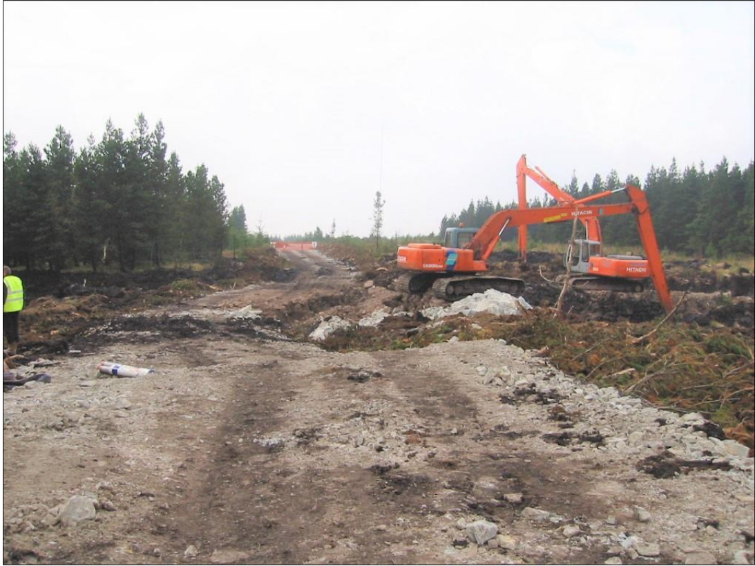
Plate 10-1: Excavation at Turbine T68 at the time of the slide
