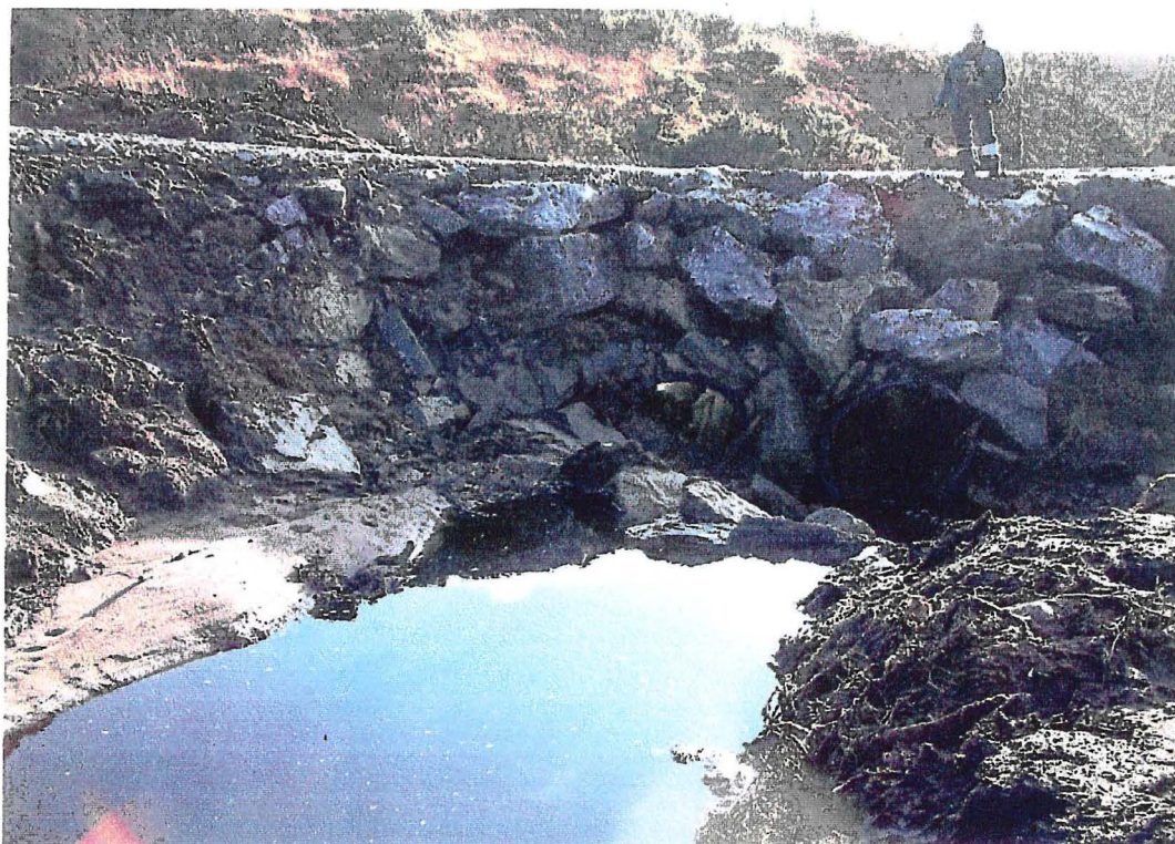
Plate 4 Chainage 198-199 the gauge of the pipes here should be increased to assist flow through.
